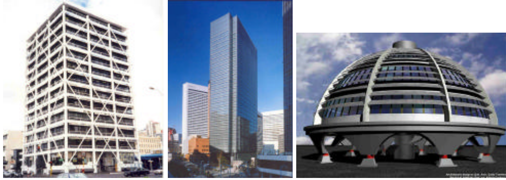
Figure 1. (a) Union House, Auckland - (b) Umeda DT Tower, Osaka - (c) Emergency Management Center, Foligno (Italy)
